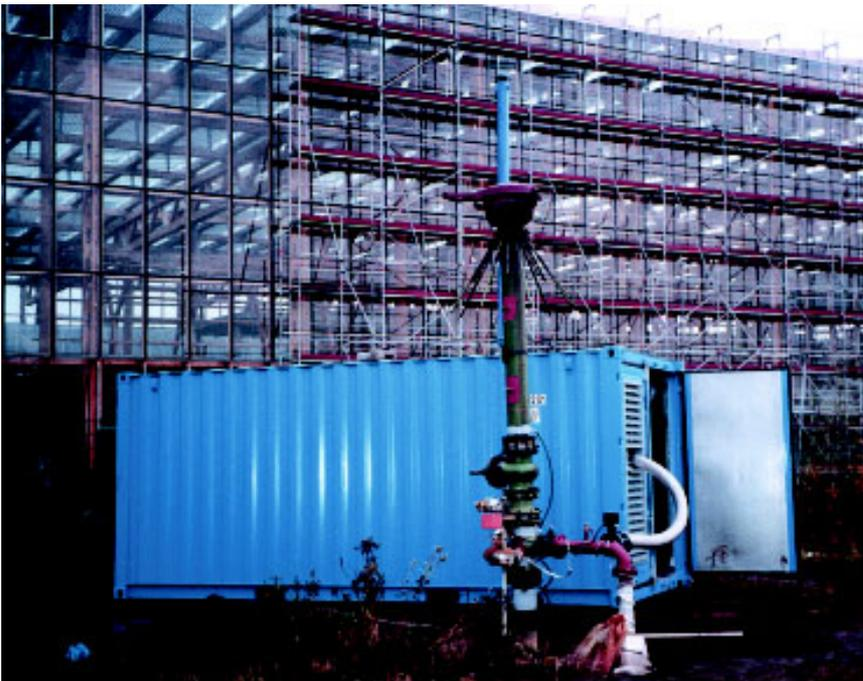
Methane gas – in the air a highly flammable and explosive mixture controlled extraction is of double use. Well-regulated energetic utilization of coal mine gas minimizes the risk and hazards by discharged methane gases.
