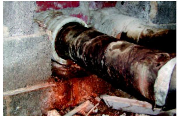
Leak in district heating pipe successfully detected using dissolved helium
